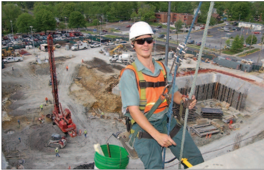
Kyle Kruckenburg, site operations manager with American National Skyline Industries, gets ready to wash windows on the 1000 wing of Boone Hospital Center. Behind him is the construction site for the new patient tower project.
