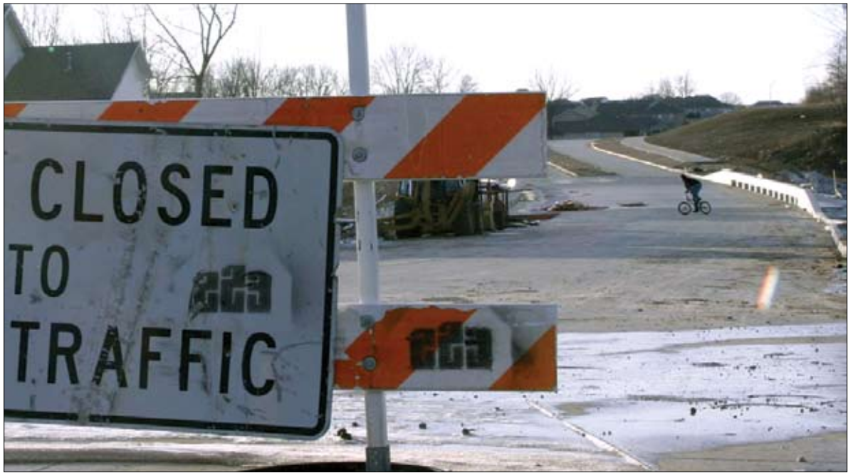
A construction project that will widen Scott Boulevard is under way.
